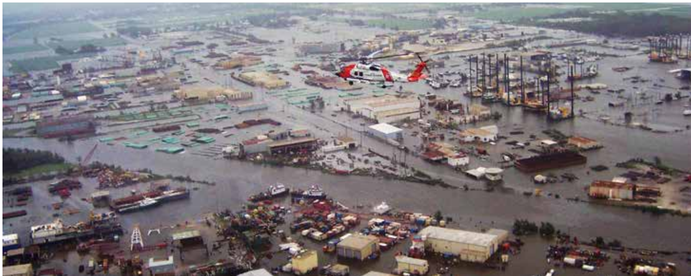
Hurricane damage, Elizabeth City, North Carolina
